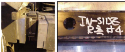
Fig. 4. Installation status and the dent defect of ball type LM guide.
